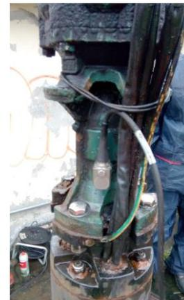
**Figure 7: vibration accelerometer installation on a 45 kW submersible well pump in a Publiacqua groundwater plant (Florence – Italy). The vibration of the pump is continuously monitored by the Department of Industrial Engineering of the University of Bologna, with the final aim to perform CBM strategy.**
